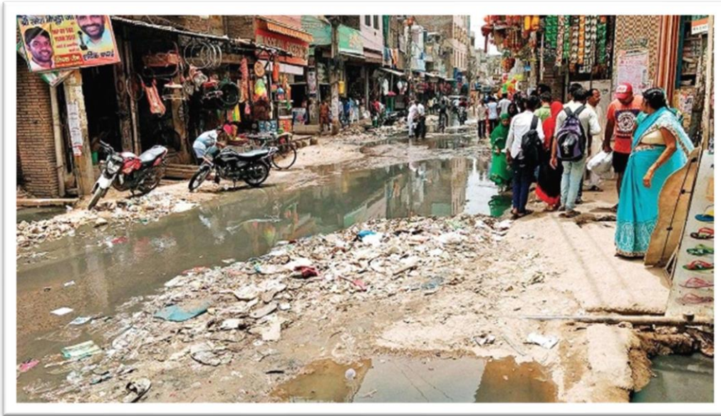
Fig. 1: Sewage collecting in open lanes in Sangam Vihar
